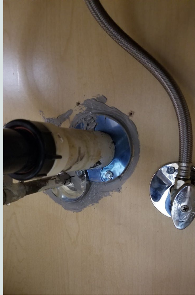
Install escutcheon plates around pipes and seal with caulking
